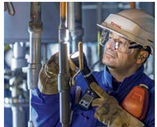
Normandy refinery in Harfleur, France.
